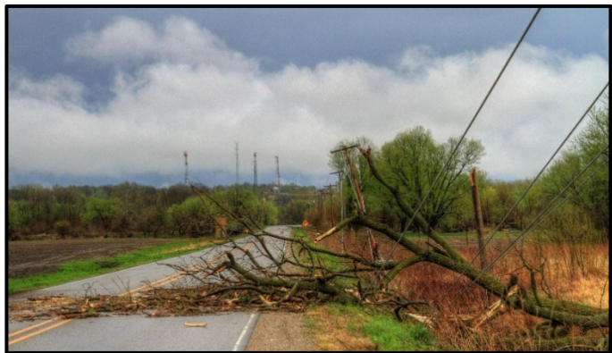
Figure 4.18. Straight-line winds toppled this dead tree into a power line and onto the adjacent county road.
